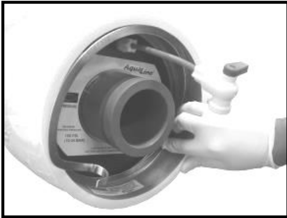
Fixing the Retaining Ring into the Groove
