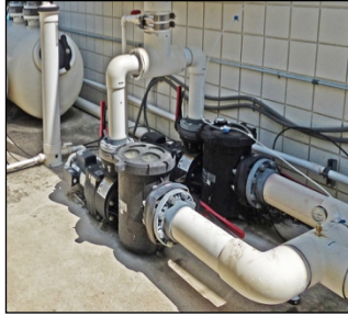
Photo 2: Dual pump system
