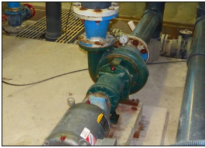
Photo 1: Single pump system
