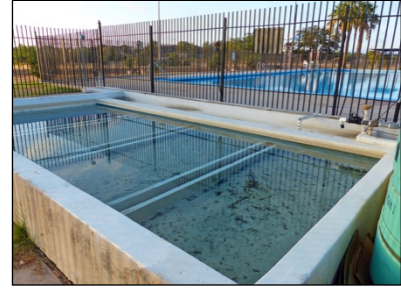
Photo 3: Gravity filter system
