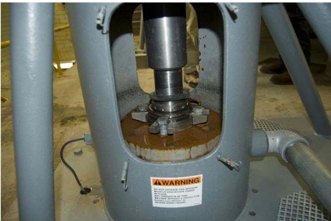
Applying a mechanical seal to a vertical turbine pump is not as simple as just switching out the packing box. There are many aspects of the installation to consider.
