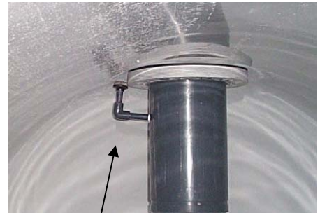
Automatic Air Relief Assembly
