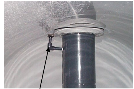
Automatic Air Relief Assembly
