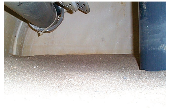
Above: Sandbed should be flat and smooth when sand is installed.
