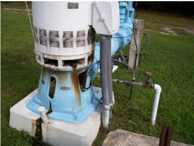
*Note the pressurized prelube line (to the right) going to the discharge head.*
