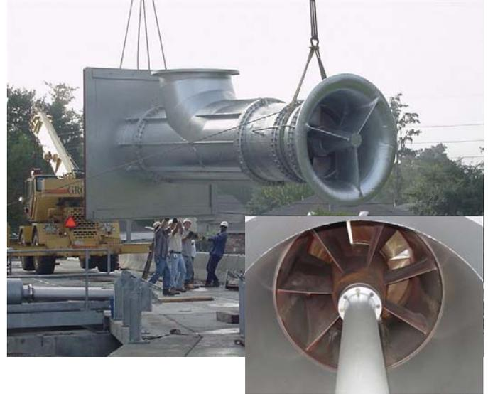
Many propeller pumps are used for drainage or flood control. Parson & Sanderson, who have represented Verti-Line for decades in Louisiana, sold two model 54P's. A new design for Verti-Line, they were driven by a diesel engine via right angle gear. These pumps help protect Ormond subdivision in Destrahan, LA, which is part of St. Charles Parish. Pictures courtesy of Jeff Leedy at Parson & Sanderson.
