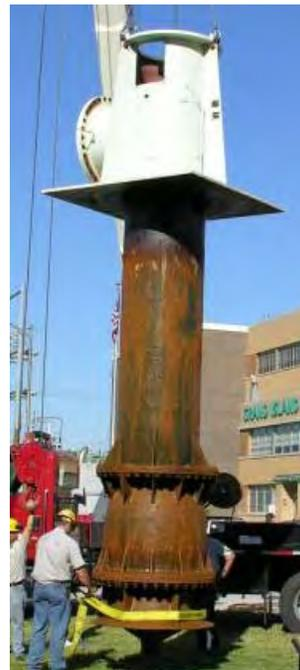
A phone call later, I was in touch with Larry Keown, Plant Superintendent for the City of Grand Island Burdick Station. Larry confirmed that the old Verti-Line's were still in operation for the power plant's cooling towers. Originally installed in September, 1971, these 46FHL single stage units are rated for 20,700 gpm @ 66.4 ft TDH. The pumps are driven by 450 HP motors turning 505 rpm at full load.
