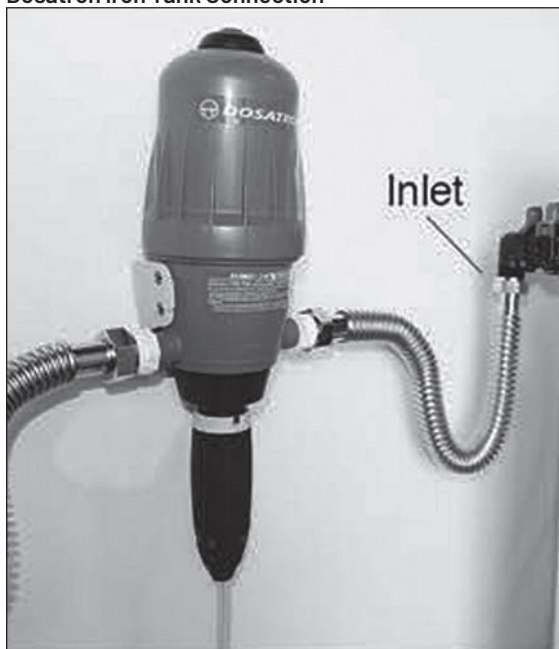
Dosatron Iron Tank Connection
