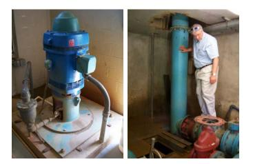
**Campbell County, VA** 15EH – 2 stage 2,100 GPM @ 129' 100 HP @ 1800 RPM Below Ground Discharge Sold by Wood Equipment Company Tom Callahan of Wood Equipment is standing next to the below ground discharge piping. If you have a pump installation you'd like to share, send us a picture! Please include a brief description of the pump, service, and location. All submissions will receive a free gift from our Company Store.
