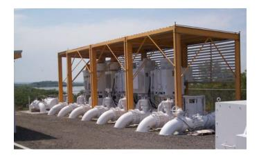
The river intake booster station has a line of seven 2000 HP Verti-Line 30KL – 5 stage turbines, each rated for 11,000 GPM @ 605' TDH. Six pumps run full bore throughout the summer, averaging 92 MGD.
