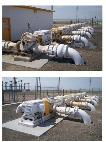
The third booster station has ten 350 HP Aurora 10x12x18 411-BF split case pumps, each rated 6000 GPM (*a*) 190' TDH. This station distributes water to various pivots as well as feeding a fourth booster station which has eight 700 HP Aurora 12x14x18 split case pumps, each rated 8,135 GPM (*a*) 292' TDH.
