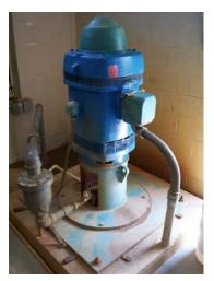
the pump revealed bronze shavings. most likely from a worn packing box bushing running dry startup. at Though the ARV looked big enough, was plugged. it This pump a good example of the damage caused by not evacuating air fast enough.
