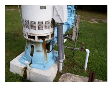
Note the pressurized prelube line (to the right) going to the discharge head.
